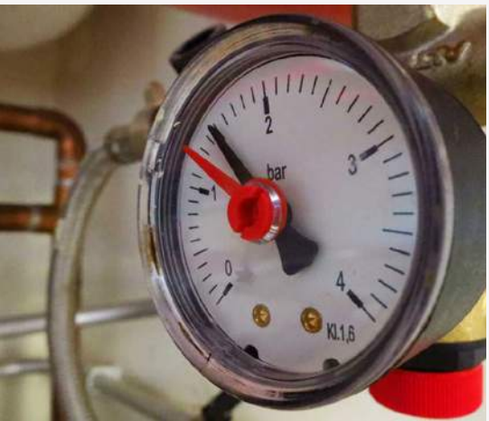
PRESSURE GAUGE SET TO 1.5 BAR
